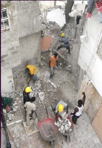
Workers hard at work demolishing St. Joseph's.
